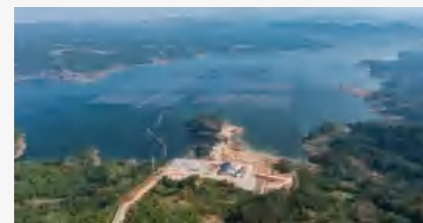
Cirata Floating PV Project
