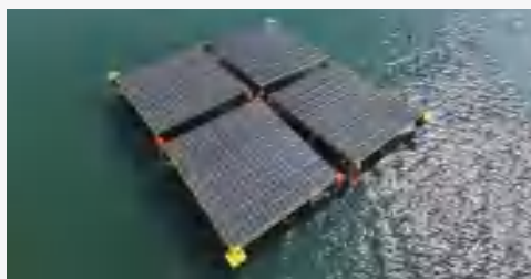
Semi-Submersible Offshore Floating PV Project
